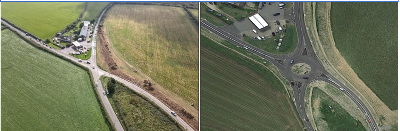
Figure 26 Lynton Cross safety improvements, with crossroads upgraded to a roundabout
