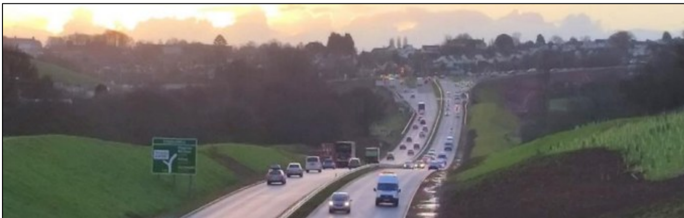
Figure 17 South Devon Highway completed scheme
