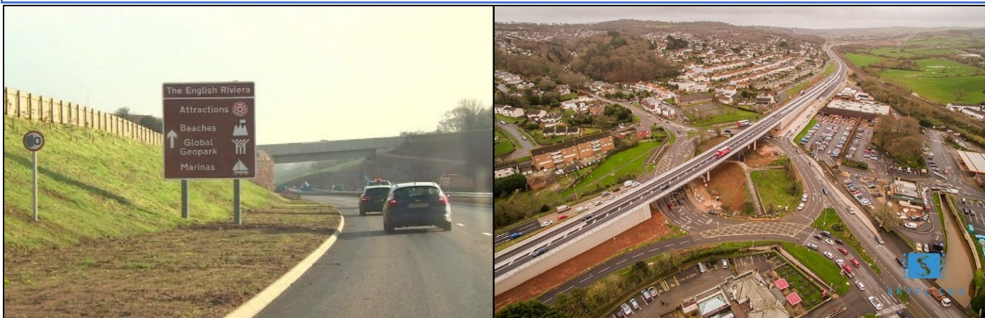
Figure 7 South Devon Highway including flyover of Penn Inn roundabout
